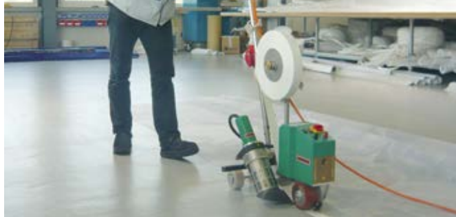
Welding tape at maximum speed.
